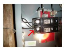
Breaker Amp Rating 100 / Normal for California construction, Appears
