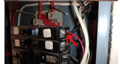
Two wires garage sub panel - NTBS
