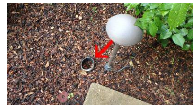
Missing drain cover drain clogged
