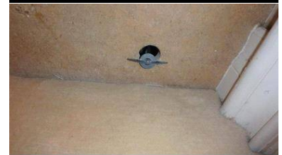
missing gas cover sleeve
